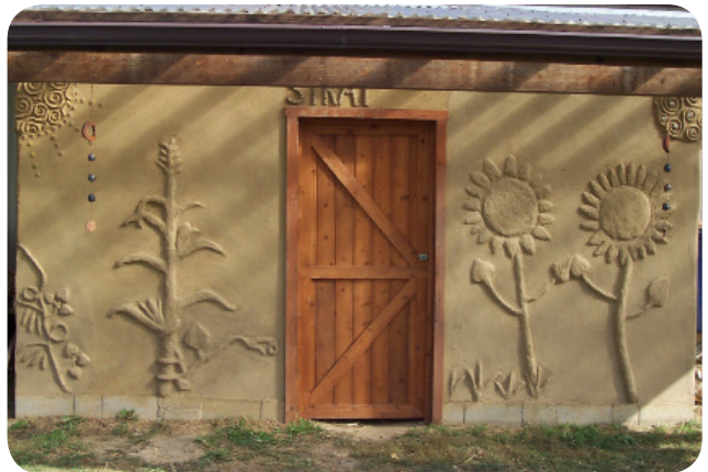
"Summer" side of Stratford's straw-bale garden shed; almost completed
