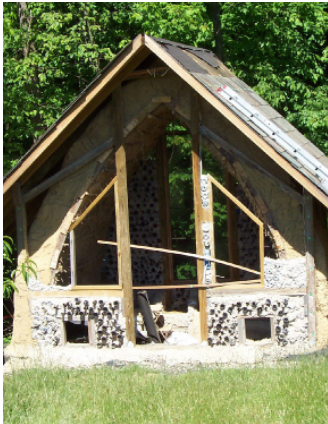
A cob/bottle chicken house under construction at Blue Rock Station in Ohio
